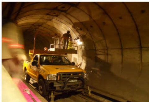
Figure 2. Installing the measuring section for tunnel monitoring
