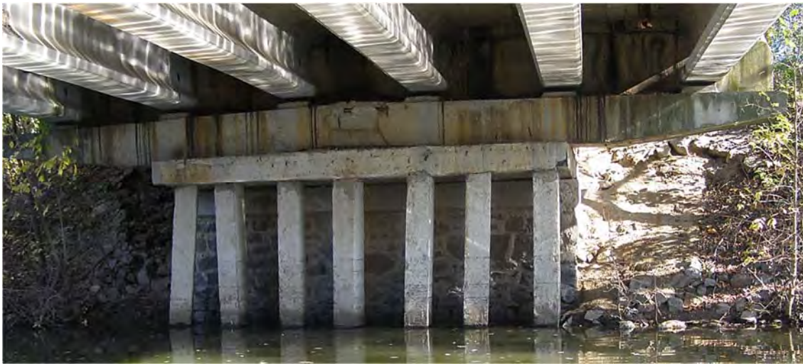
Figure 1 – Example of a typical crossbar system (constant height) of a beam bridge, where the pile foundations perform the function of the shaft of the bridge abutment
