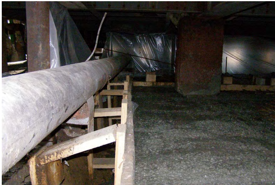
Figure 2 – The stage of concreting the foundation slab is strengthened without the use of vibration.
