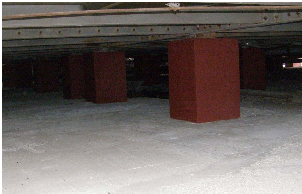
Figure 3 –The finished construction of foundation reinforcement.
