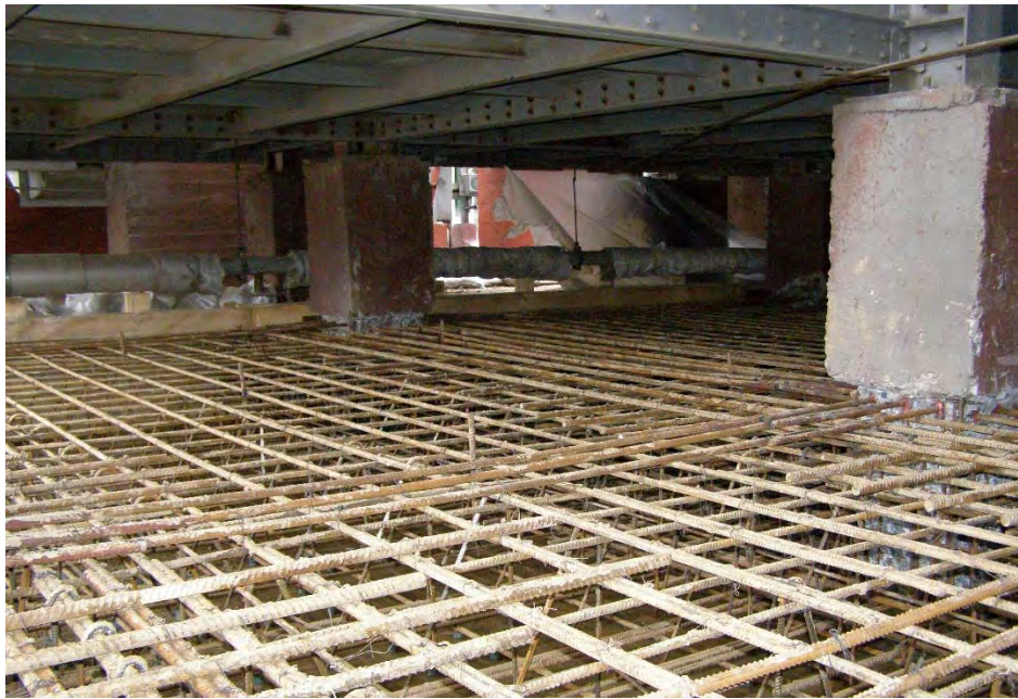
Figure 1 – The stage of installation of reinforcing frames of the slab of reinforcement of the foundations of the furnace
